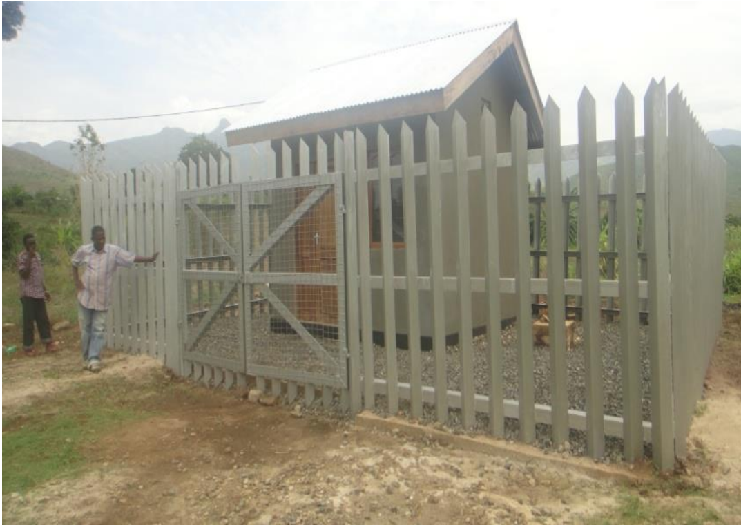
Figure 4.20: Constructed pumping scheme house
