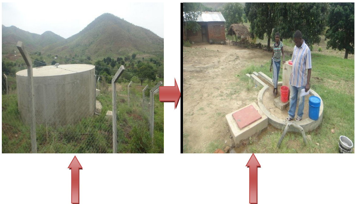
Figure 4.19: Storage water tank at Gudugudu hamlet in Mlali village (left) and Community water point (right) .
