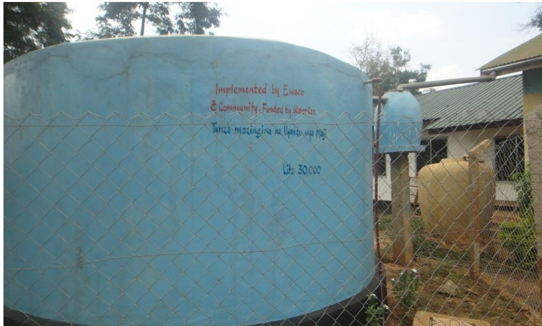
Figure 4.10: Rain water harvesting system at Mlali Heath Centre
