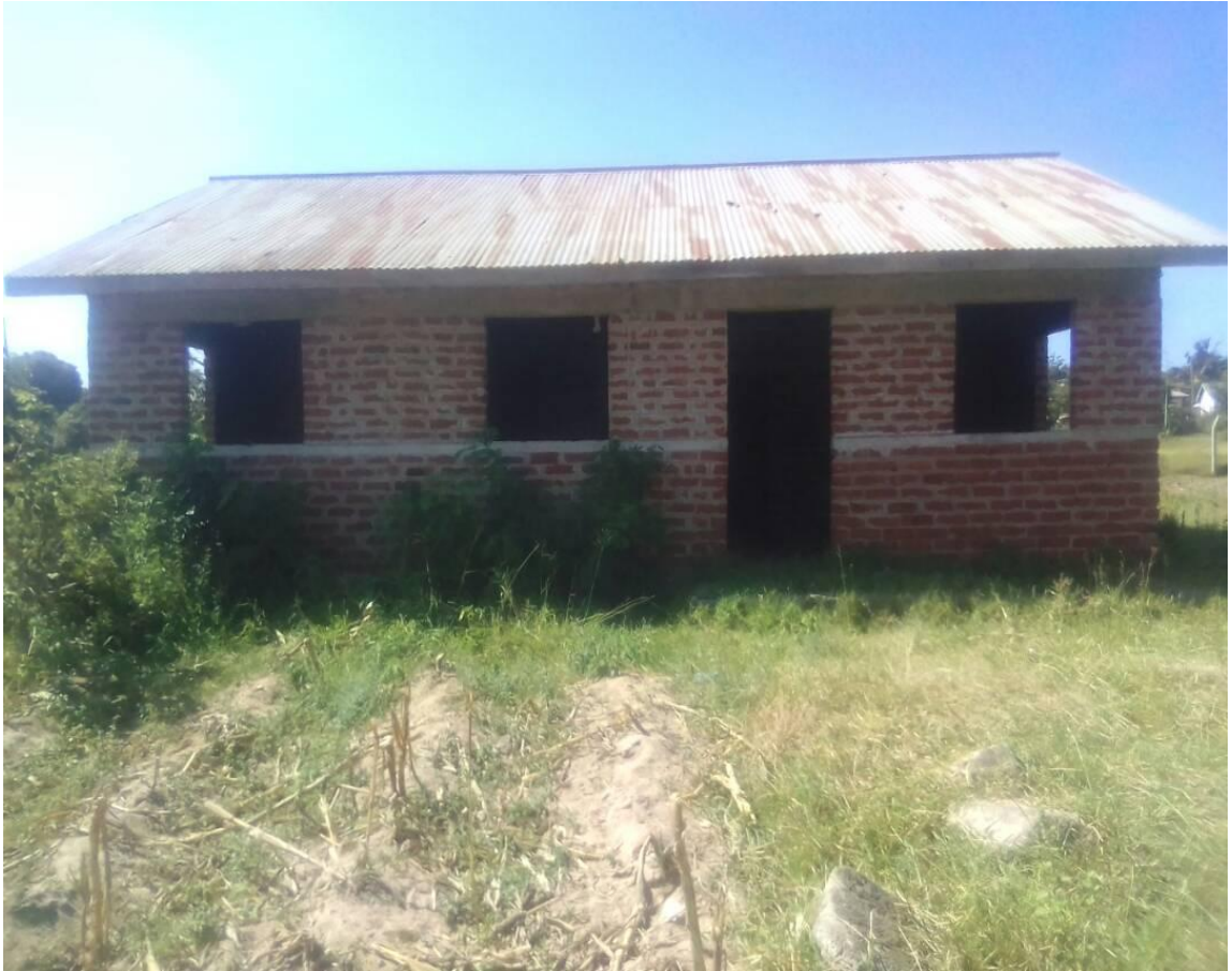
Figure 4.2: Unfinished teacher's house within Ilemela Municipality
