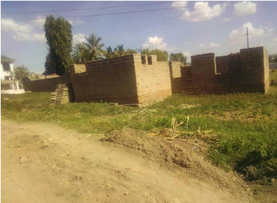
Figure 4.1: Unfinished police station building within Ilemela Municipality
