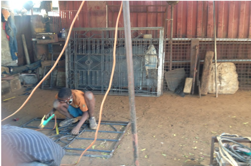
Figure 4. 2: Weldingoperator at Gerezani, Ilala operating with improper working facilities.
