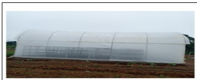
Figure 1. Solar Dryer House
