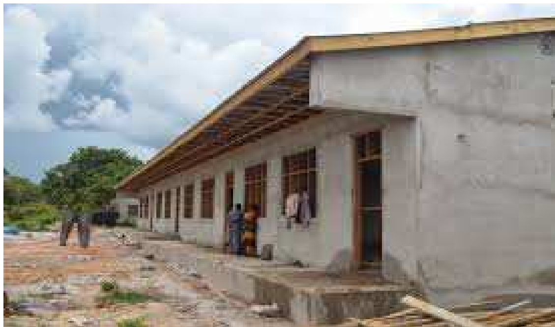
Figure 4.4: Construction of four classrooms at Mchikichini ward
