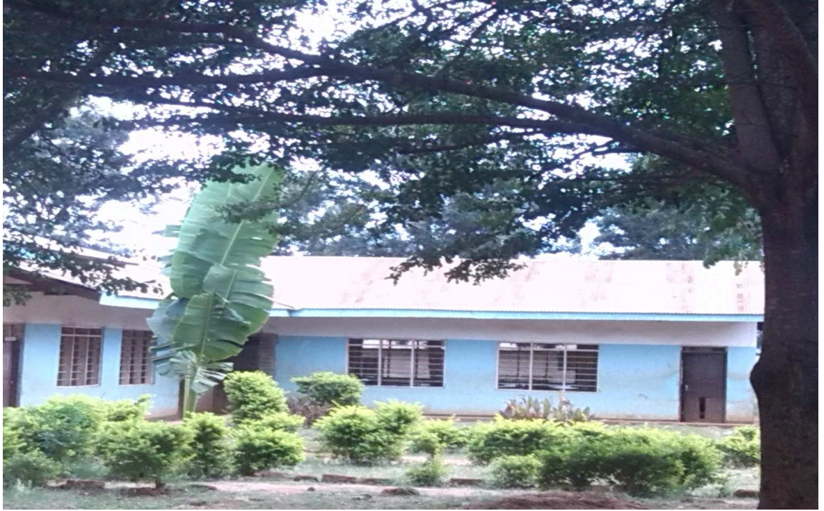
Figure 4.2: Classroom built by government at Kinyerezi primary school
