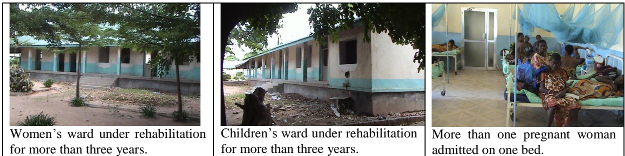
Figure 5.1: Absconded Projects at Tabora Regional Hospital.
