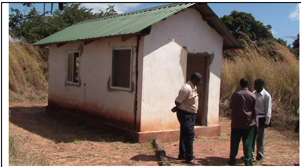
The Regional Inspection Team at Kitunda HC.
