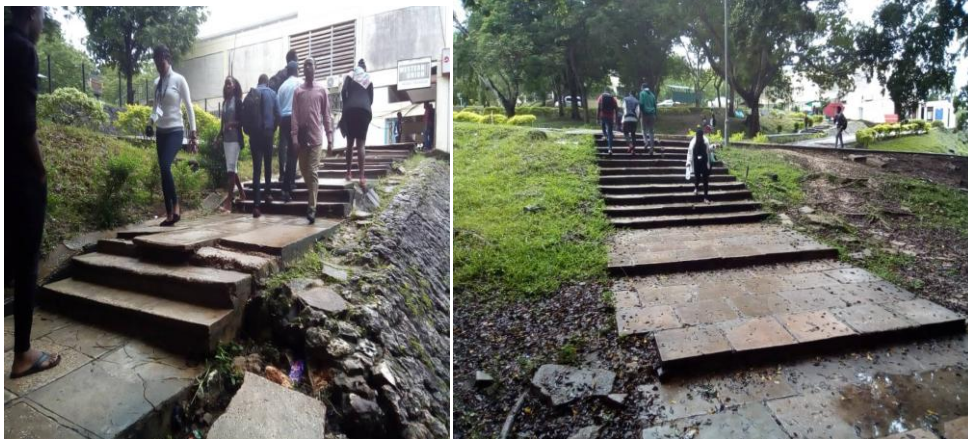
Plate 4. 2: Stairs from the academic bridge to the Postal office, cafeteria and hostels
