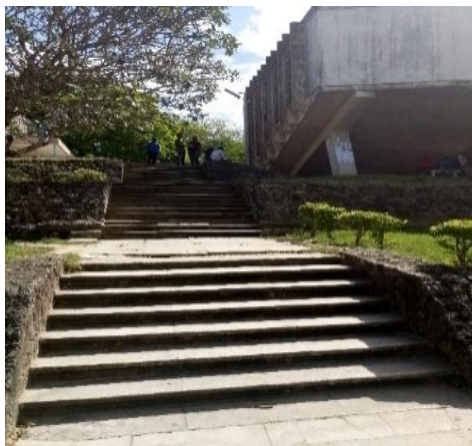
Plate 4.9: Unsupportive building structures for VIS at UDSM
