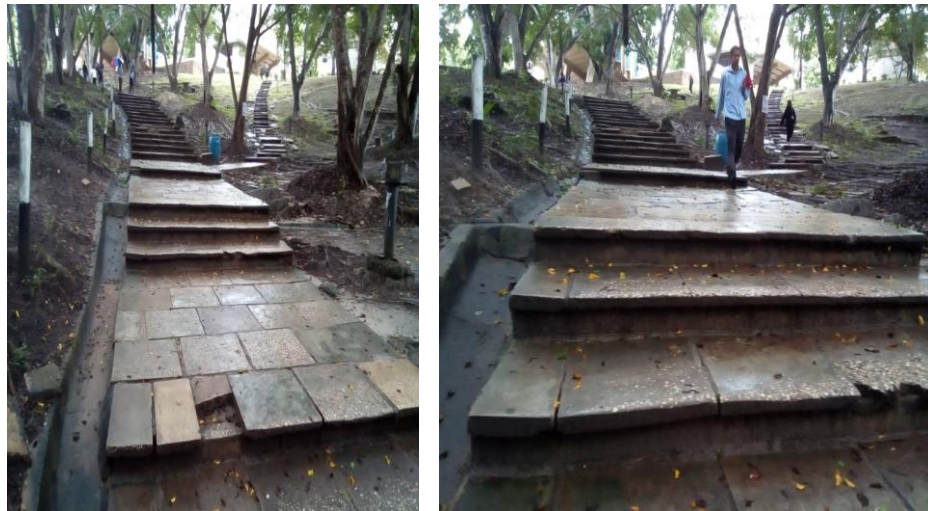
Plate 4.1: Stairs from the academic bridge to IRA, main Library and lecture rooms
