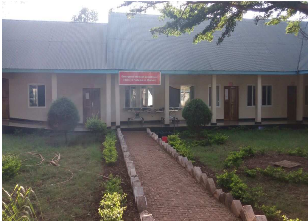
Figure 4.1: Emergency Unit building funded by Geita Gold Mine
