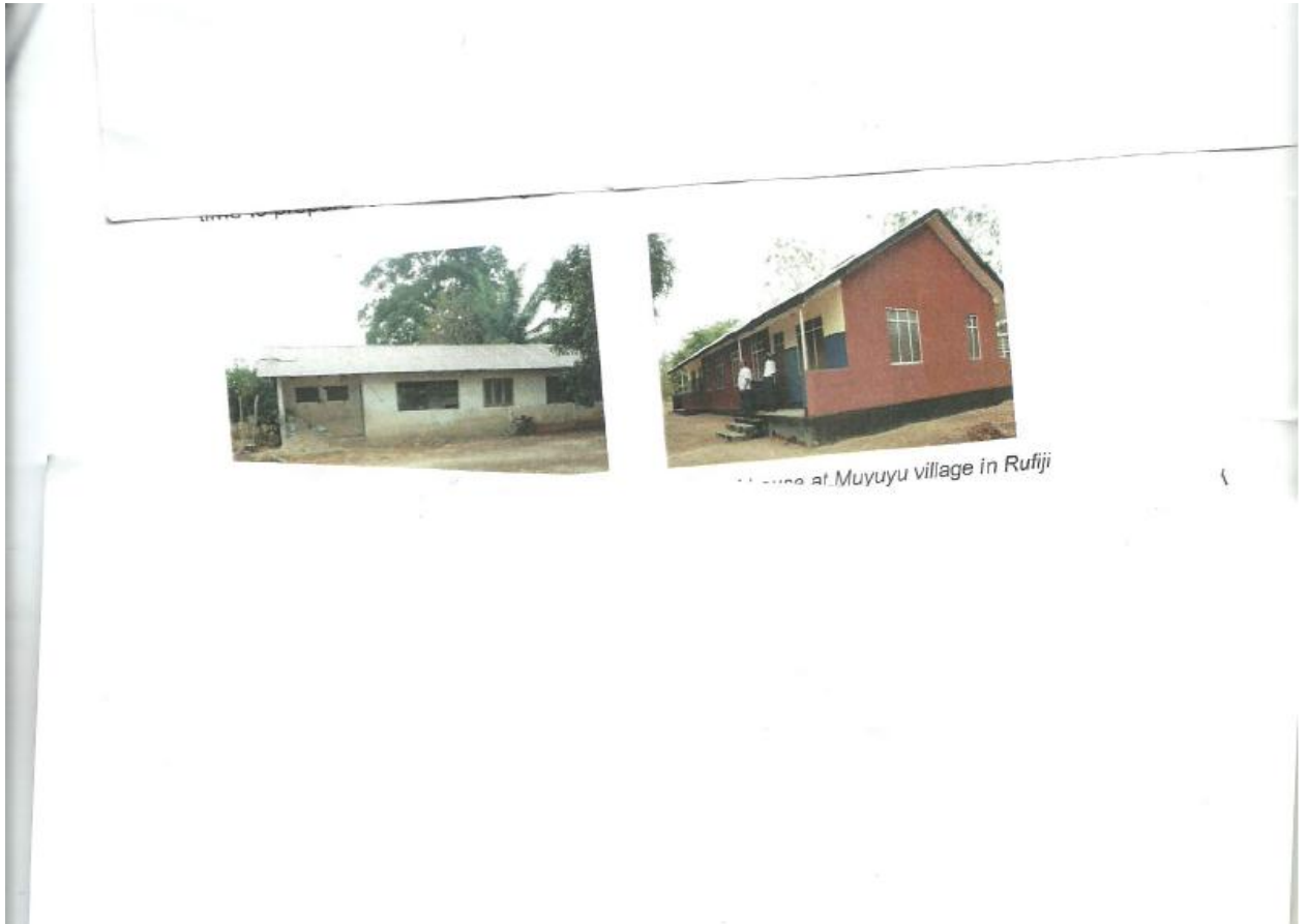
Figure 4.3 Teachers houses constructed by Songas
