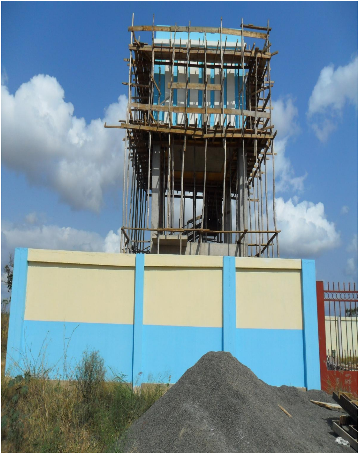
New constructed water tank as an extension of the project
