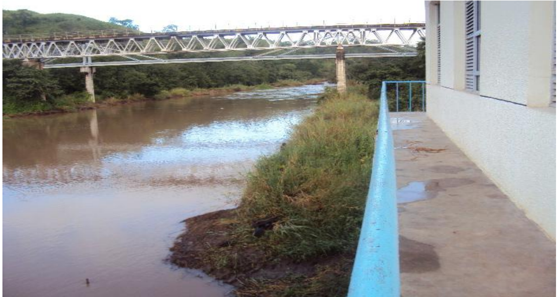
Figure 3.1 Shows the Source of Chalinze Water Supply Project near Wami Bridge
