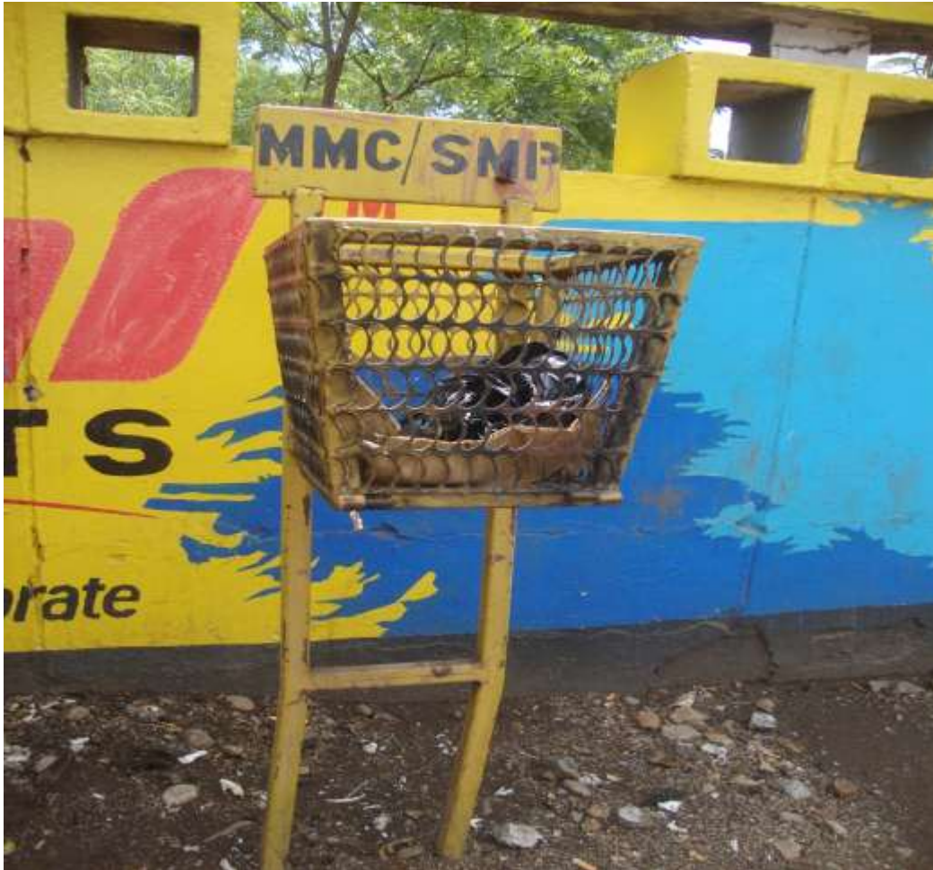
Figure 4.17: Showing one of the remaining roadside dustbin in Mawenzi ward
