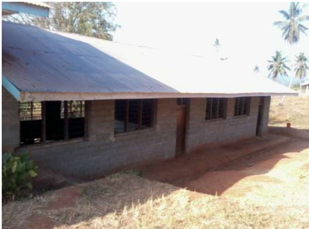
Figure 4.5: Unfinished classroom building constructed by the Community at Masimbani village
