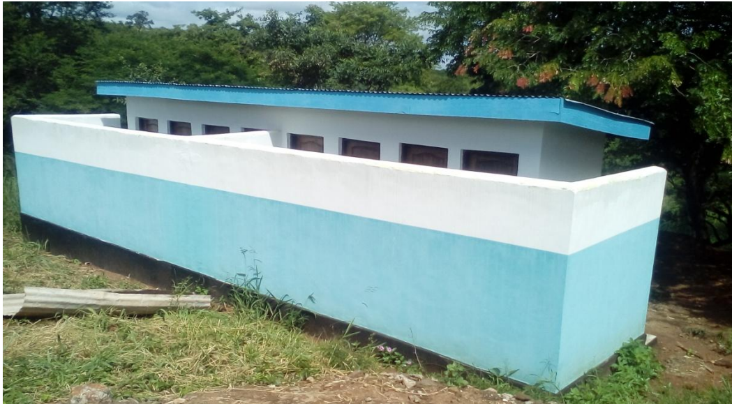
Figure 4.5 Toilet building at Kiroka secondary
