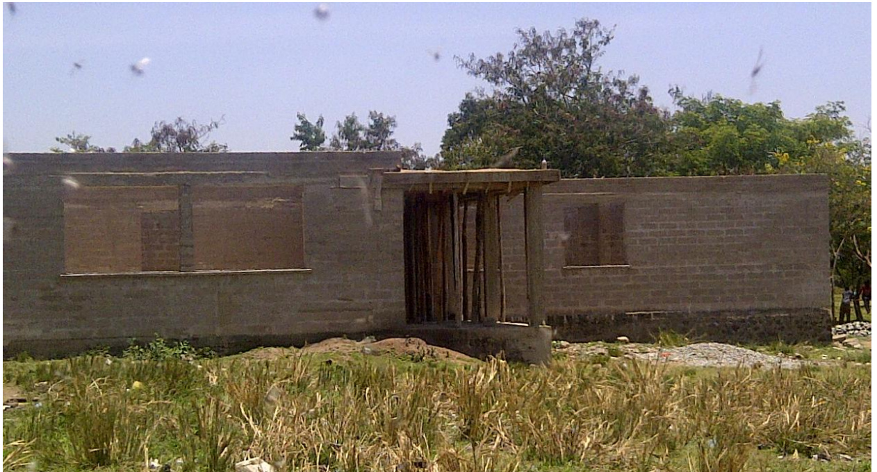
Figure 4.14: Nyamongo Primary Court (under construction)
