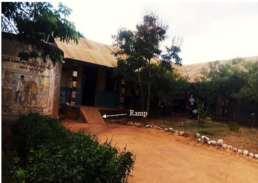
Figure 4.4 Picture indicating classrooms with ramps
