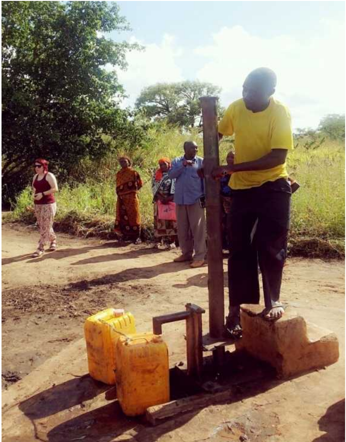
Figure 4.12: Maintenance of hand pumped shallow well at Mafuru village
