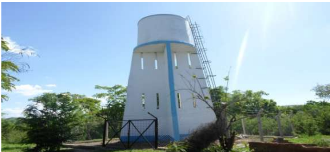
Figure 4.4: Water tank after project in Dalla village
