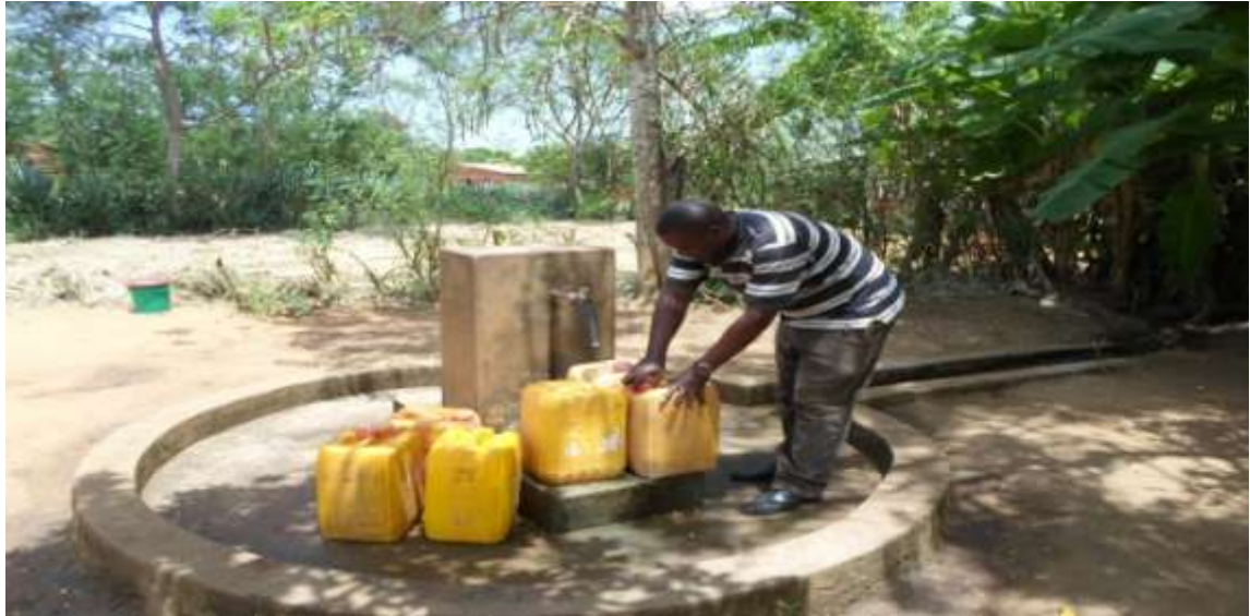
Figure 4.2: Public Water point of Mkambarani village
