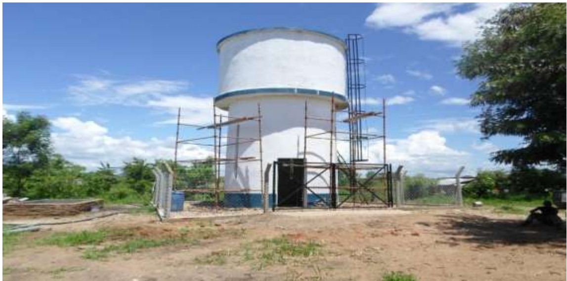
Figure 4.7: Construction of water tank in Mvuha village
