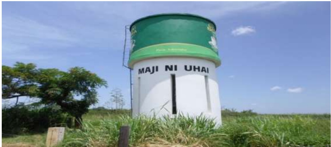
Figure 4.1: Water tank after project in Mkambarani village
