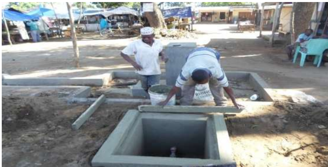
Figure 4.8: Water point construction in Mvuha village
