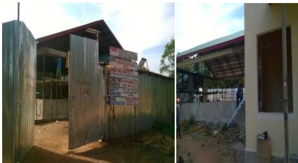
Figure 4.3: Picture 1 Construction of Farmers Horticultural Service Centre in Mlali
