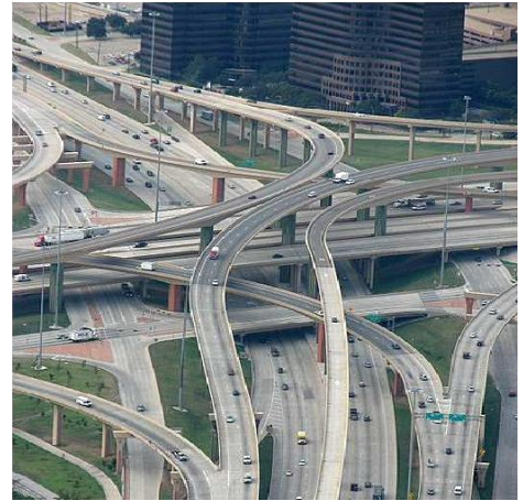
Figure 4.11: Complex grade separation
