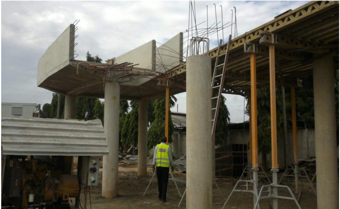
Figure 2.2: A bridge under construction at Ubungo through DART project
