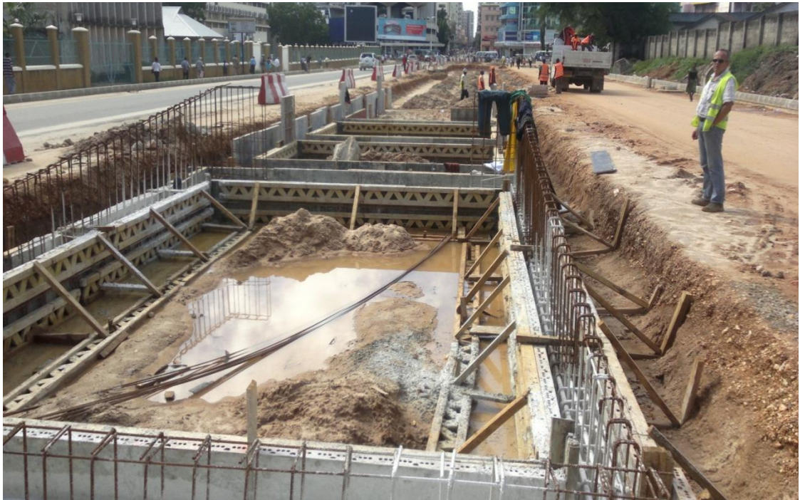
Figure 2.1 Ongoing road constructions under DART project
