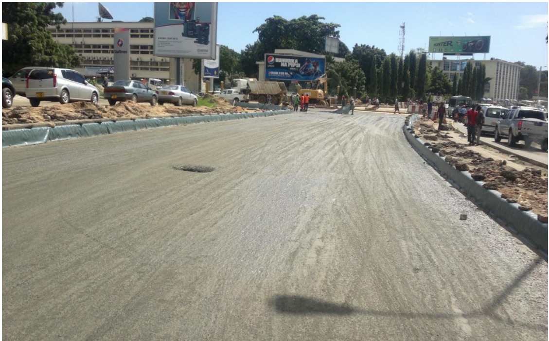
Figure 2.3: A new constructed road under DART project
