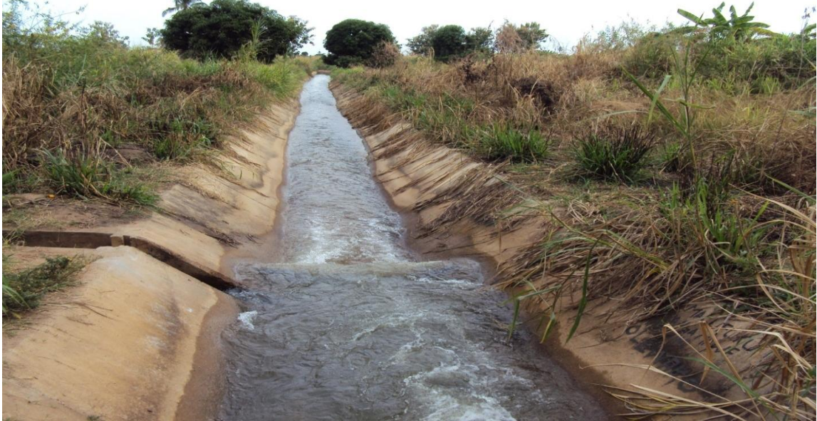
Figure 6.4: Lined canal in MIS
