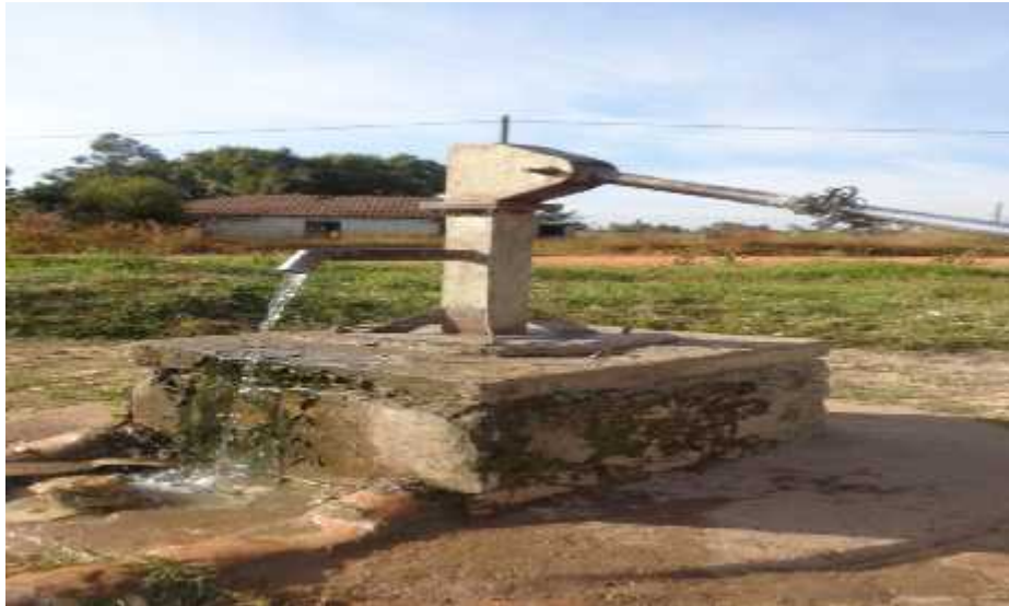
Figure 4.8: Hand pump at Kitelewasi village
