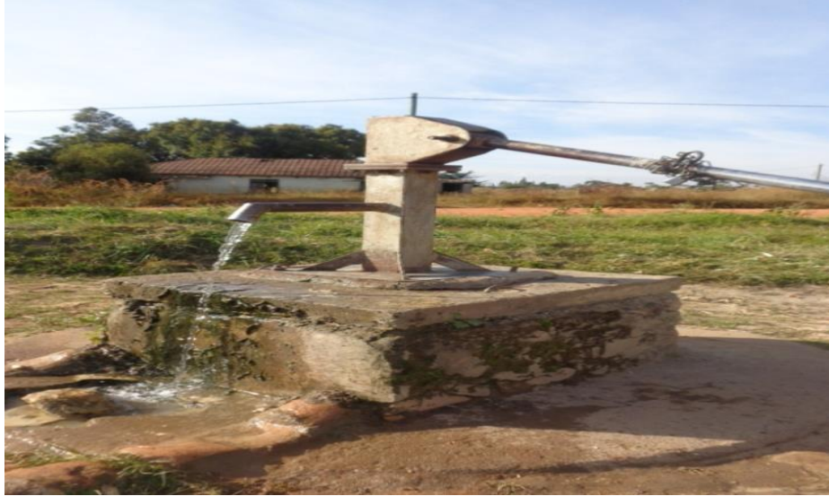
Figure 4.8: Hand pump at Kitelewasi village
