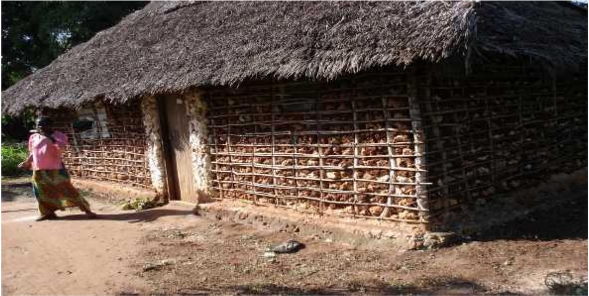
**Figure 4.8: Roof of a traditional house made by using thatches**
